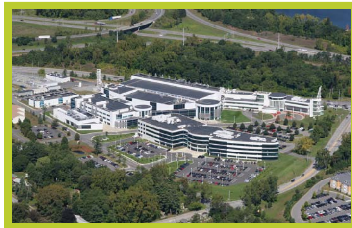
Below: The $5.5 billion Albany Nanotech Complex, 2009.
